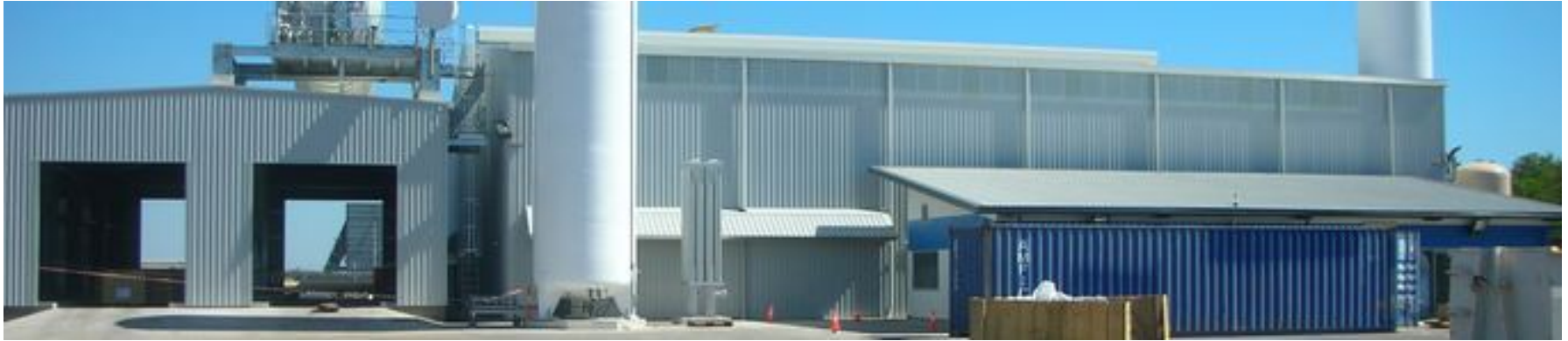
Photo: Linde/BOC Darwin LHe Plant – web sourced
